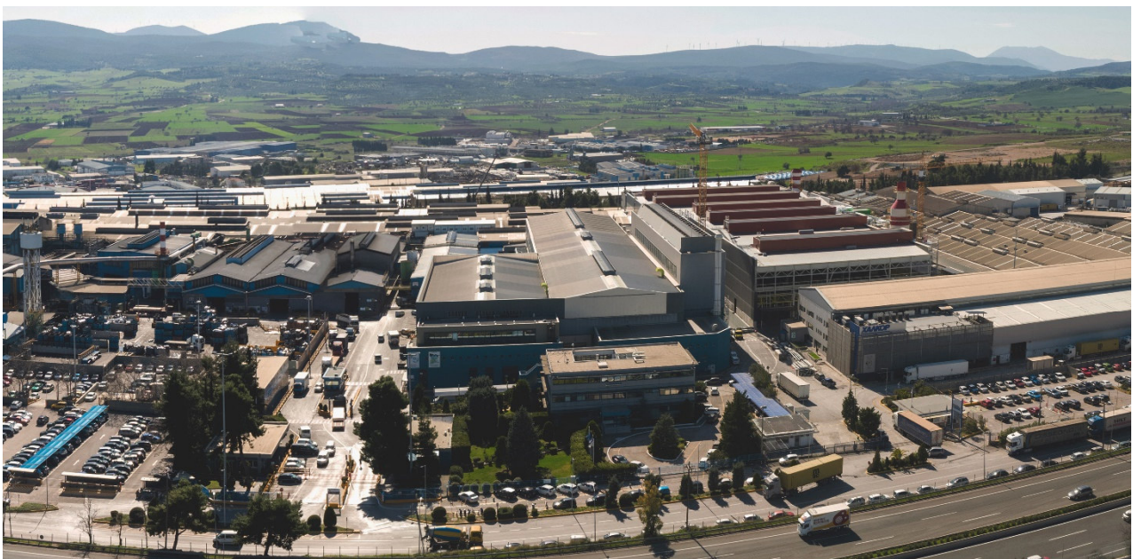
Copper tubes plant in Oinofyta, Greece - Aerial view - Photo by courtesy of ElvalHalcor
