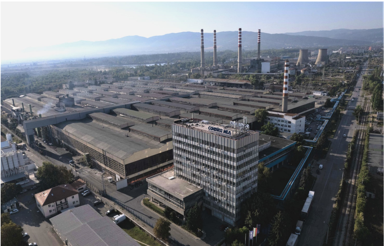
Headquarters and manufacturing plant of Sofia Med in Sofia, Bulgaria – Bird's-eye view - Photo by courtesy of ElvalHalcor
